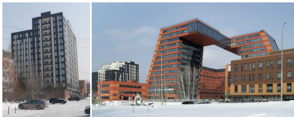
Рис. 6. Здания технопарка. Фото автора Fig. 6. Buildings of the technology park. Photo by the author
